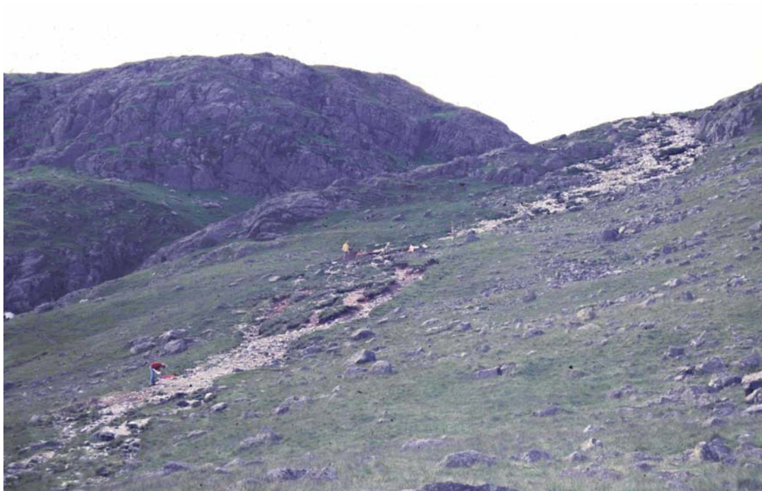
Plate 2: Harrison Path, Langdale, showing the major erosion scar up the hillside before the site was repaired with a pitched path
